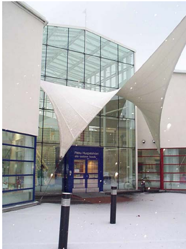
Figure 4 Point supported glass facade (in Pikku-Huopalahti, Helsinki)
